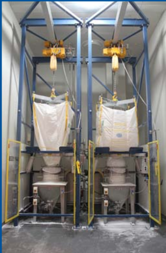
Bag unloading room, complete with 2 x "Flexicon", Bulk Bag Unloaders, each setup in a mild steel frame with electric hoist and trolley. Units complete with power cincher, bag activators, s/s hopper with agitator and vibrator. Safe working load of 1500kg, also included 2 x "Wilden" M8 Diaphragm Pumps, "DCE Vokes", dust collector and Rapid Roller Door
