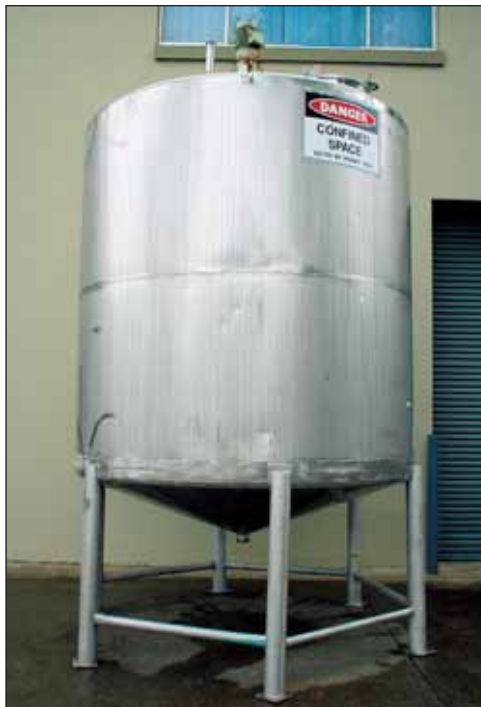
1. STAINLESS STEEL TANK
